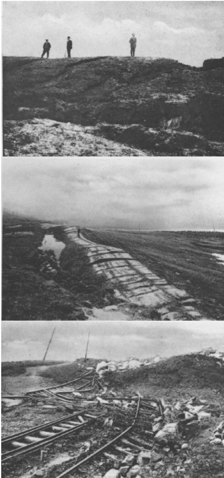
Fig. 8: Picture of the effect of the rock-fall on the alluvial, which created hills and large horizontal displacements.
